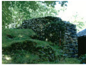
Blast walls by what was once the pressing house.
