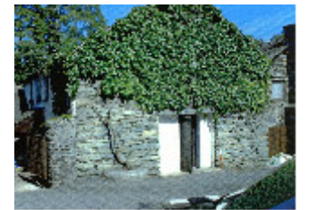
The mixing or preparing house. The column at the left was part of the wheel pit where a waterwheel would have been used to drive the mixing process.
