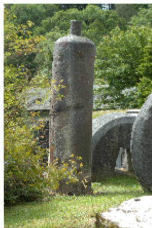
Old-style incorporating mills contributed to the closure of the Elterwater Works. Retort recently acquired from Gatebeck Mill and generously donated by Mr Brian Gregg.
