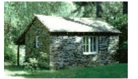
Dipping and Packing House by Hobson's Tarn.
